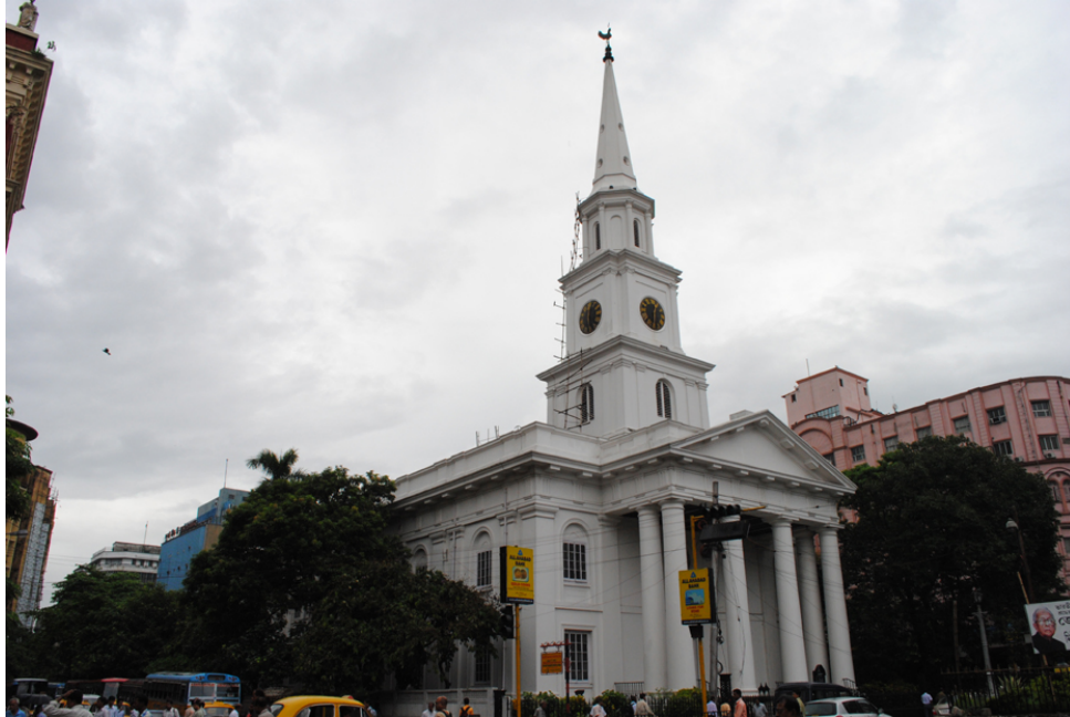
Fig.13. St. Andrews Church, Calcutta, India, Photograph Courtesy of the Calcutta.org
